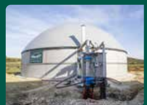
7. Day Pipeline construction completed and ready for operation
