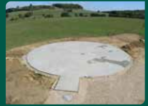
On-site base plate
